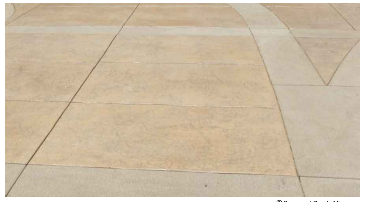
Decorative Concrete © Spragues' Ready Mix
