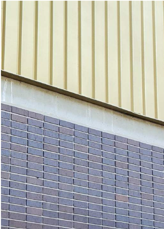
EXISTING WALL FINISHES
