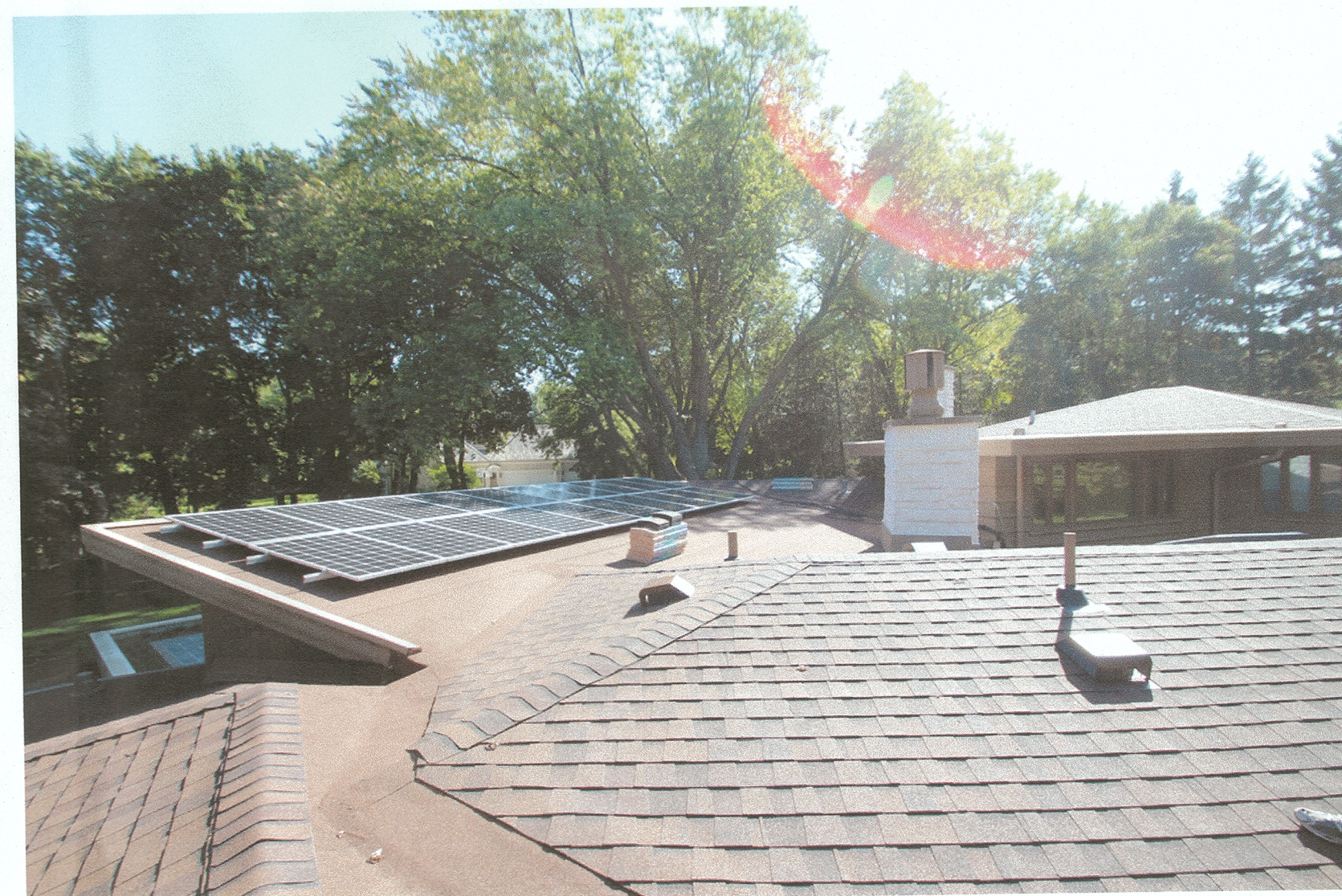
Existing roof line and solar panels (roof angles and misc. mechanical penetrations prevent more panels on roof)
