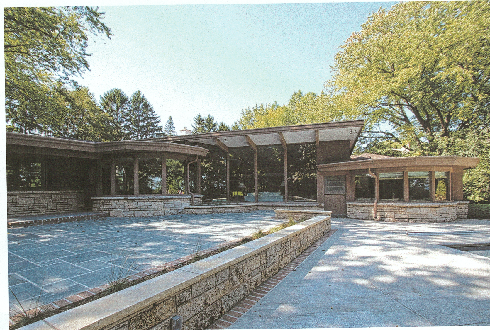
Existing house looking north close up
