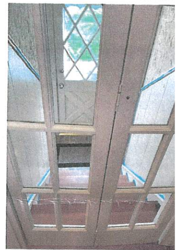
Interior Steps for Back Entrance
