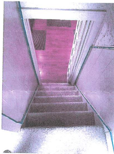
Lower Stairs from Intermediate Landing
