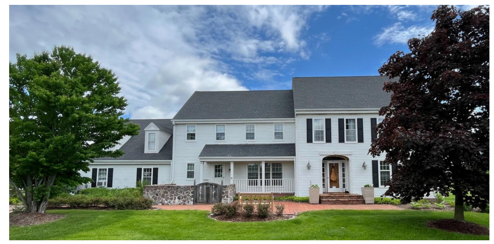
EXISTING FRONT VIEW
