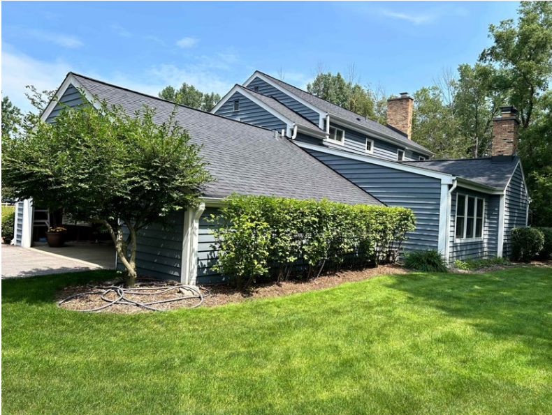
Area of expansion. Lining up new roof with adjacent roofline.
