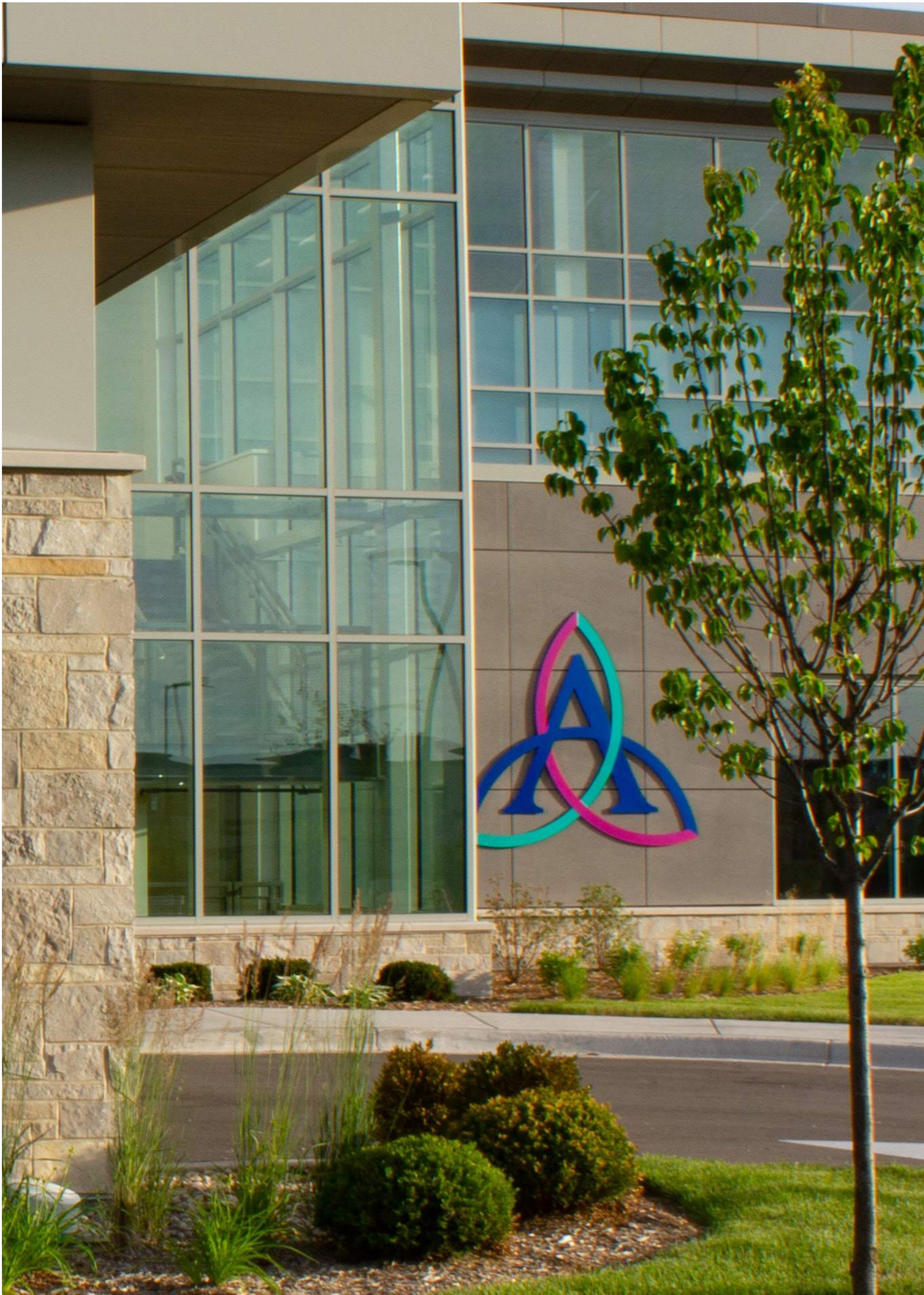
FIBER CEMENT GLASS METAL FASCIA + WINDOW FRAMES
