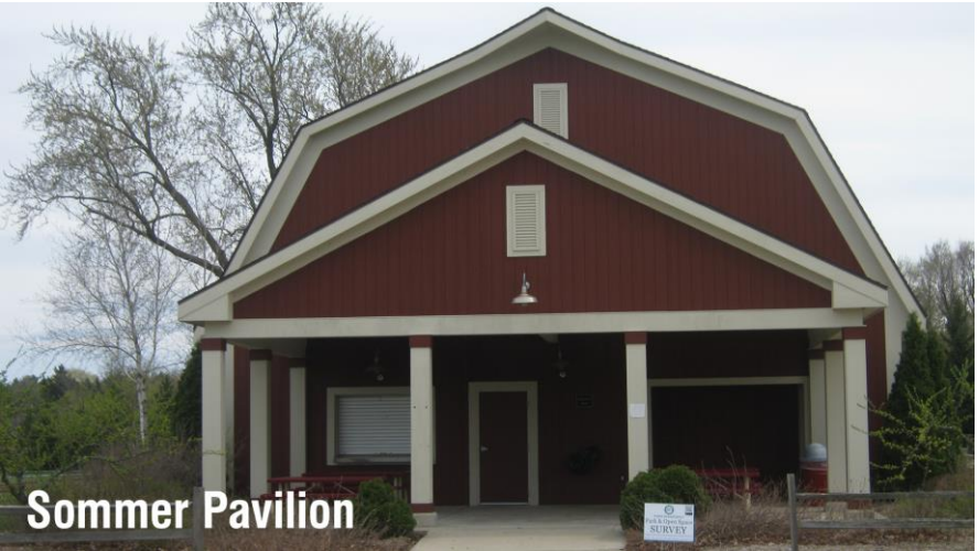
Worn safety surfacing
