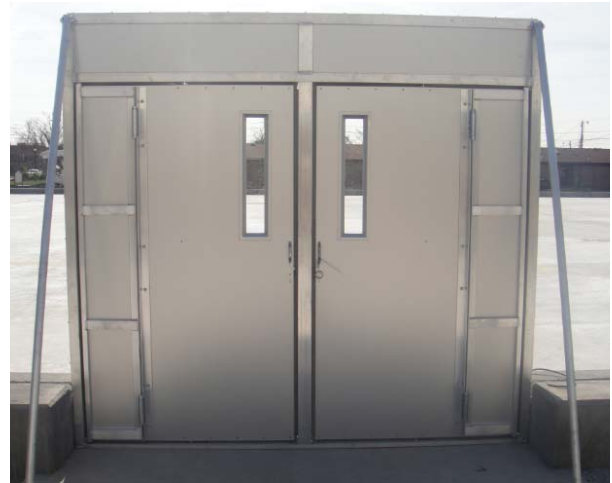
Double emergency exit door (exterior)
