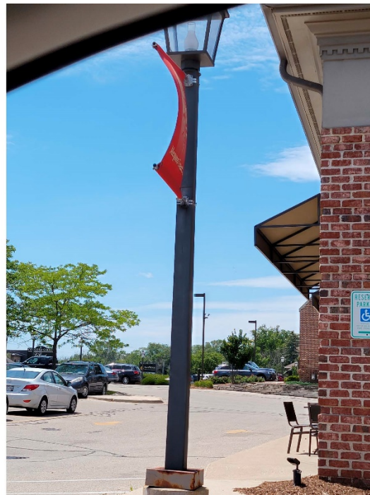
Exhibit 2: Replace or repaint parking lot lighting fixtures to address rust issues.
