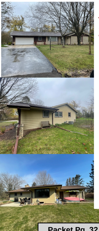
Existing Exterior Photos
