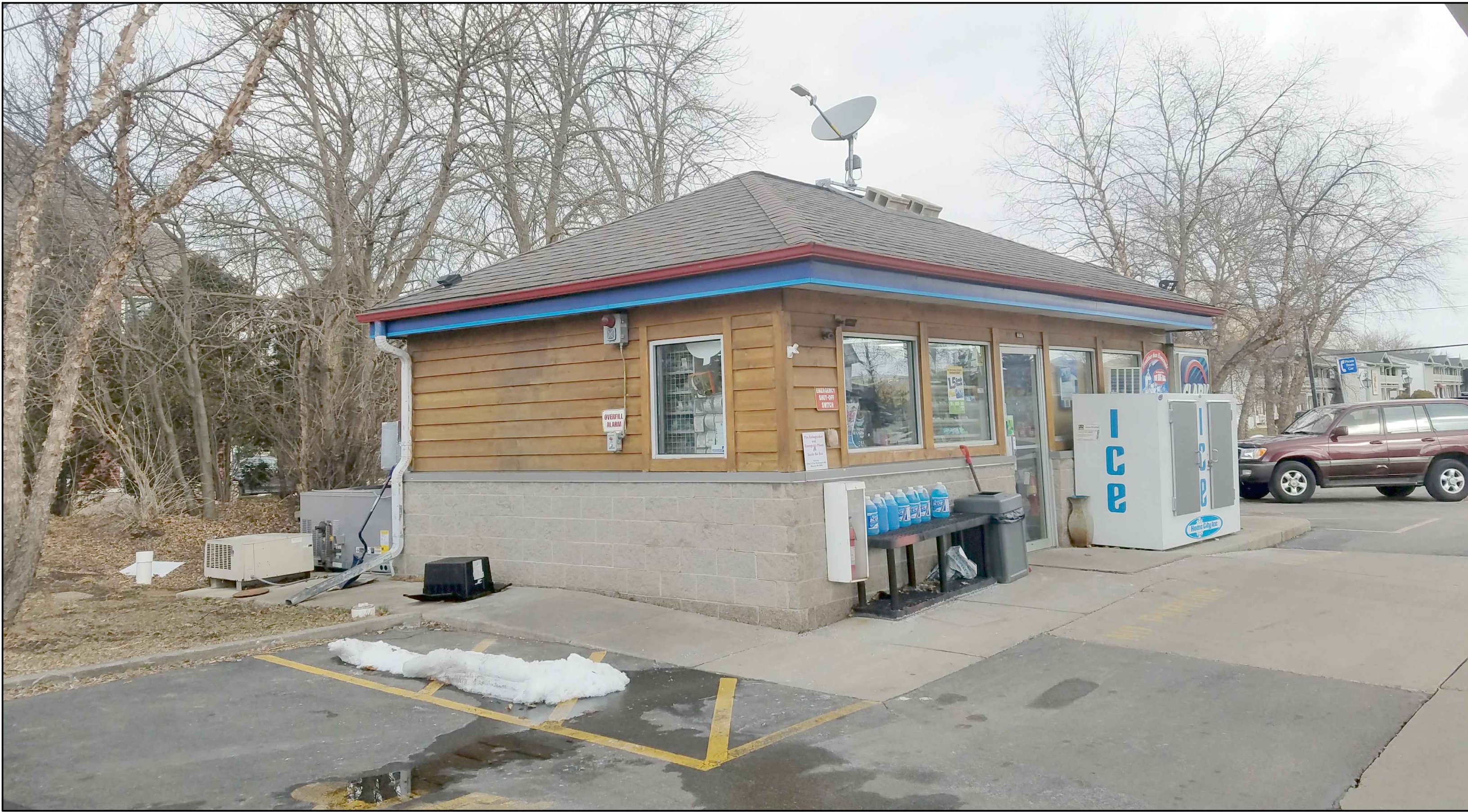
1 EXISTING PHOTO (SOUTH EAST LOOKING NORTH WEST) SCALE: N.T.S.
