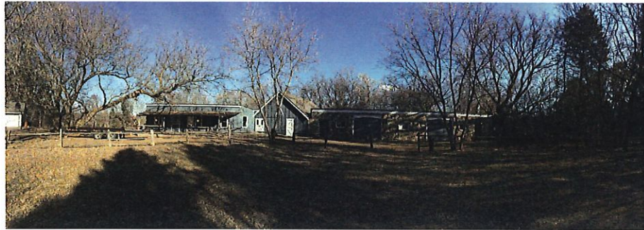
7 South Facade (full) Existing Photos nts
