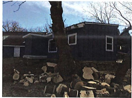
11 Reno North West (partial) Existing Photos nts
