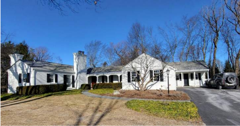
Front (South Side)
