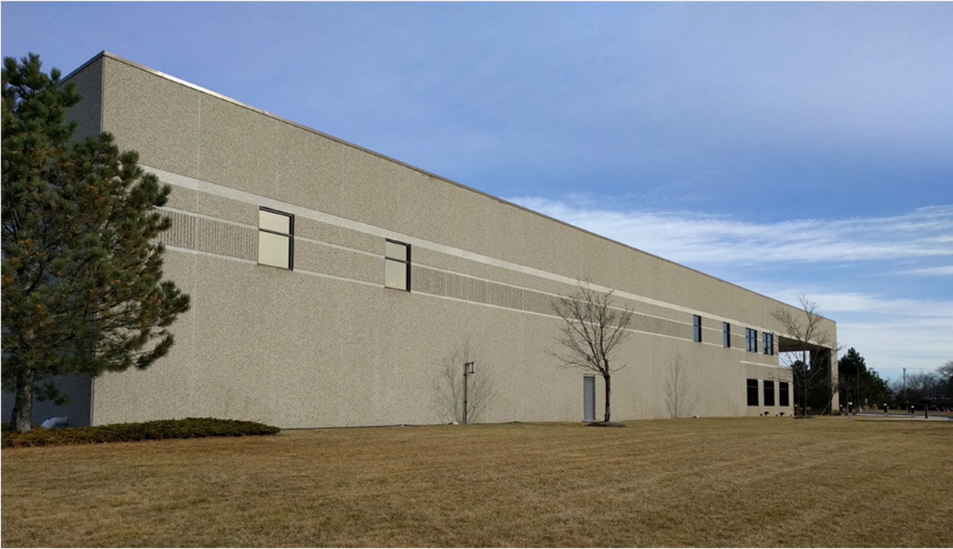
EXISTING SOUTH WALL
