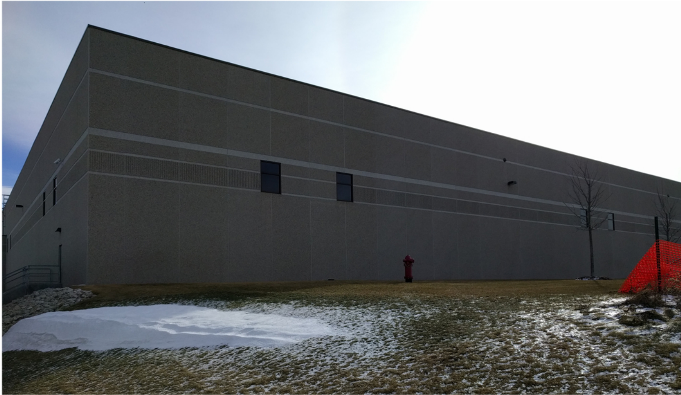
EXISTING NORTHWEST CORNER
