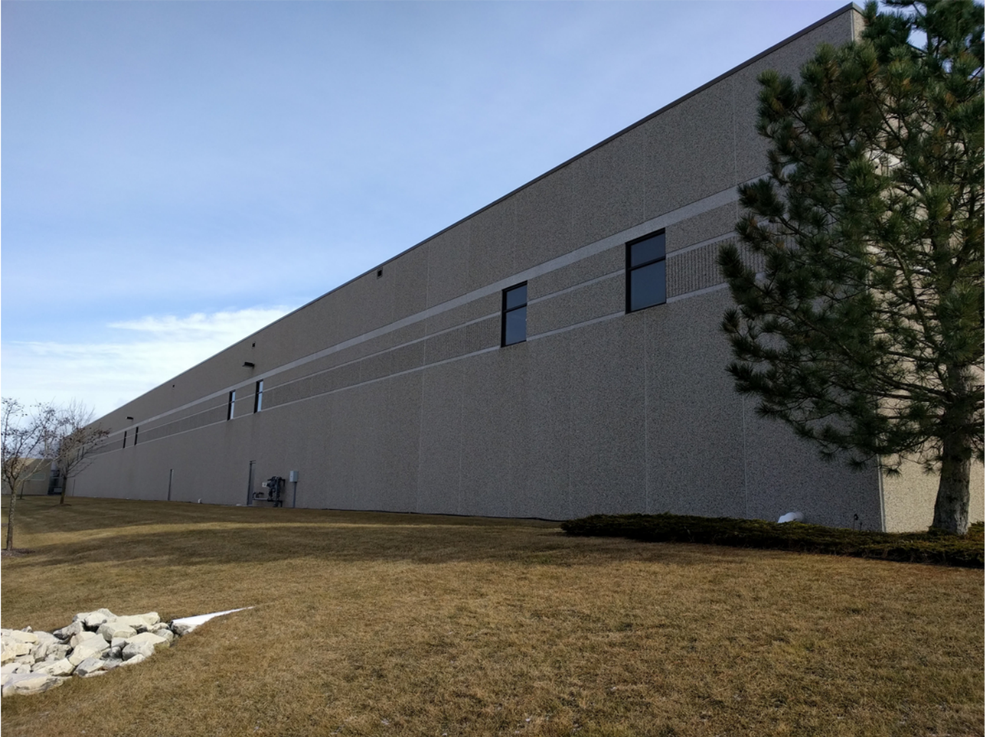
EXISTING WEST WALL
