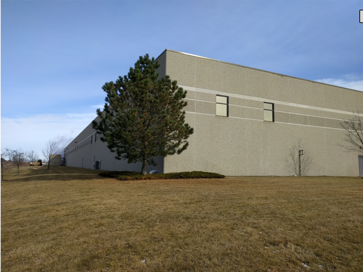
EXISTING SOUTHWEST CORNER
