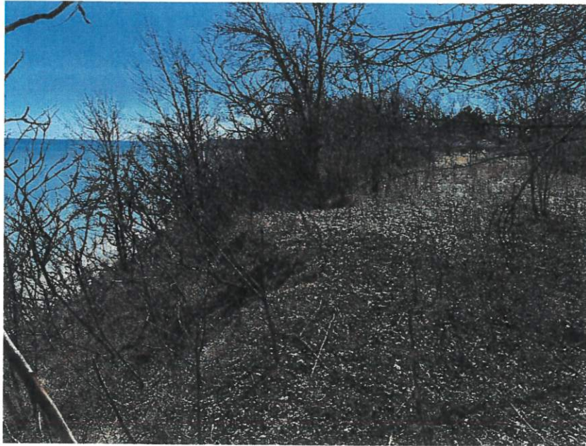
Photo 3: Looking south from the northern property boundary at the current steep scarps along the crest of the bluff.
