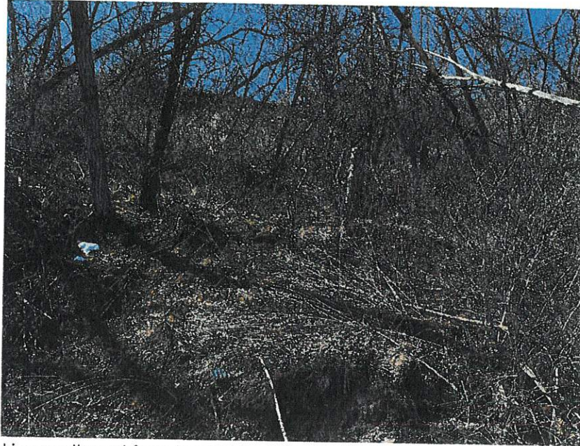
Photo 5: Looking northwest from just south of the subject property at the bluff face at the boundary between the vegetated portion of the slope and the bare portion of the slope.
