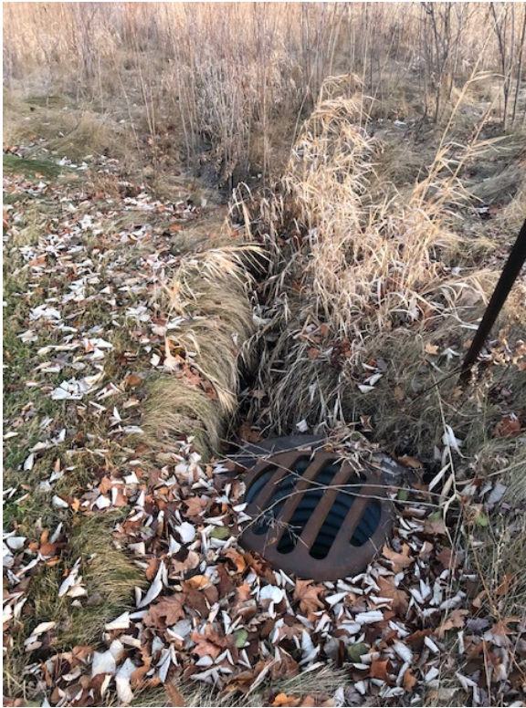
Facing north. Showing drop structure ditch that intercepts flow from the ditch.
