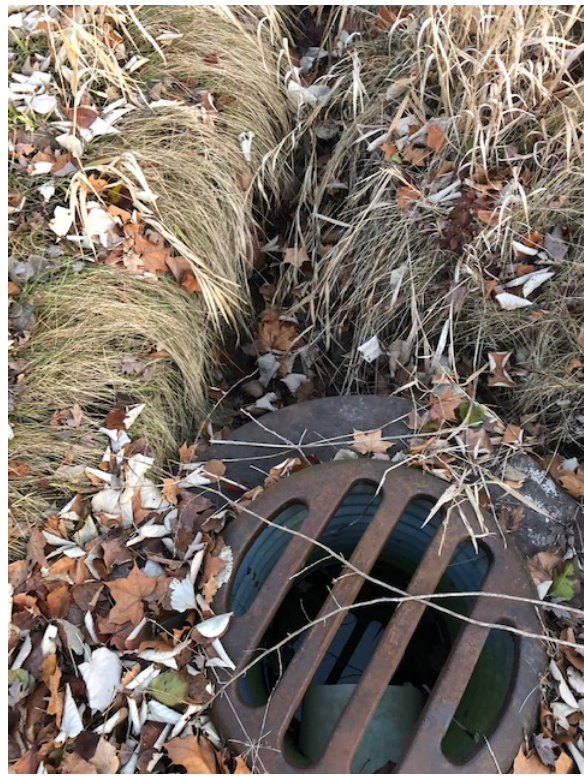
Facing north. Showing drop structure ditch that intercepts flow from the ditch.
