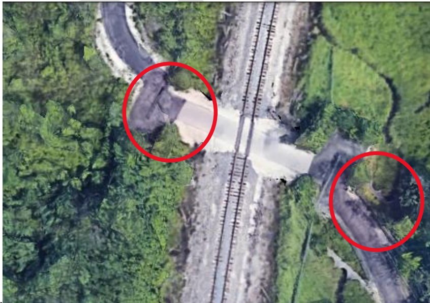
Aerial photo of crossing from Google Earth 5-24-2014
